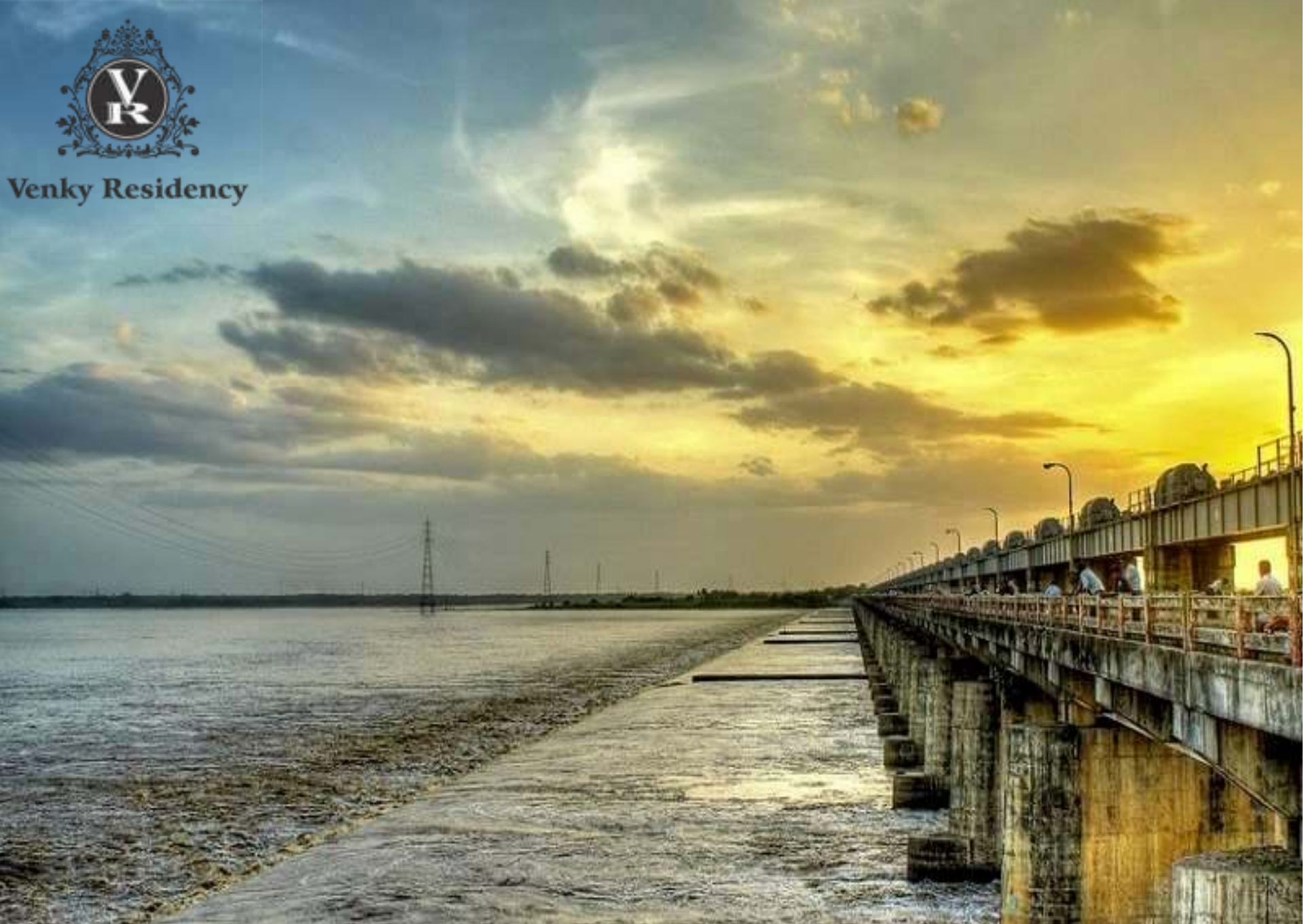
Dowleshwaram barrage built by Sir Cotton as part of aincut project that stands to this day
